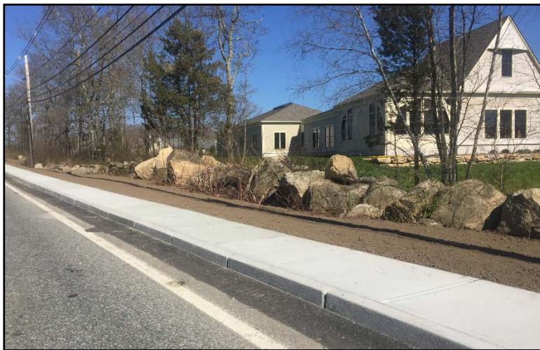
New sidewalk along Bulgarmarsh Road
