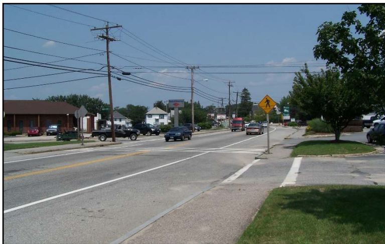
Main Road in north Tiverton is the location of many retail businesses
