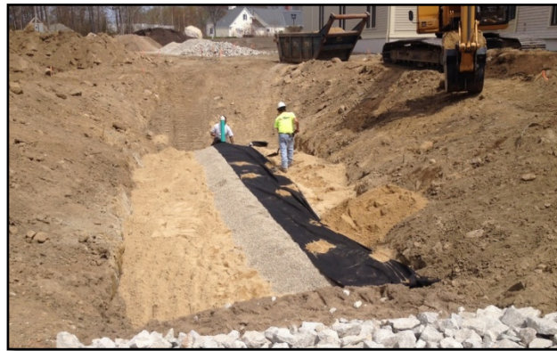
Bio-retention drainage system installation
