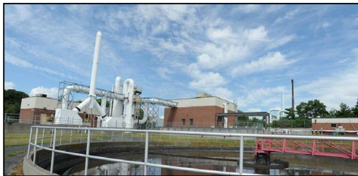
Fall River Wastewater Treatment Plant
