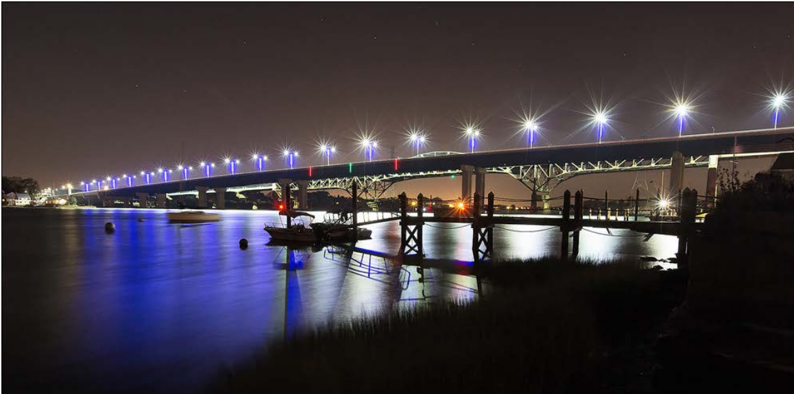
Sakonnet River Bridge
